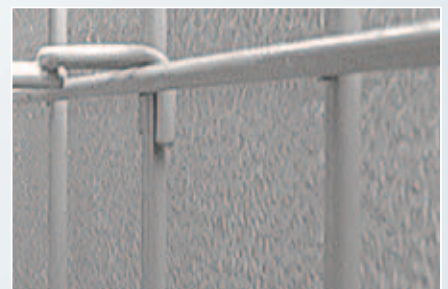
3.) Frost-free inner wall after the defrosting process
